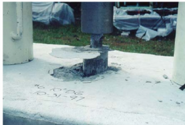
FIGURE 13 Bond Release of Concrete of Grout
