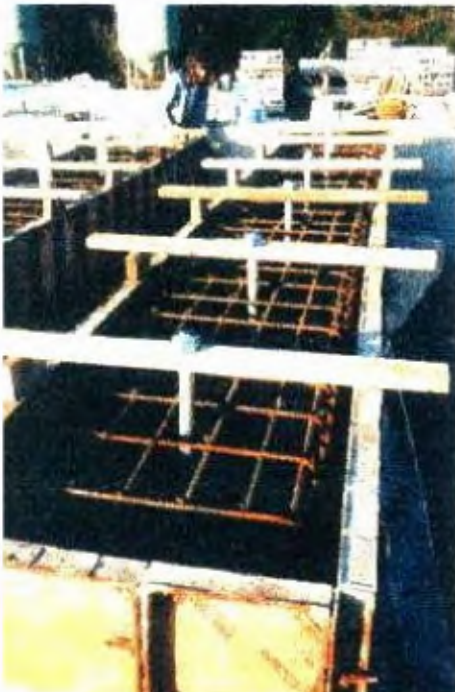
FIGURE 2 Cast in Place Bolts
