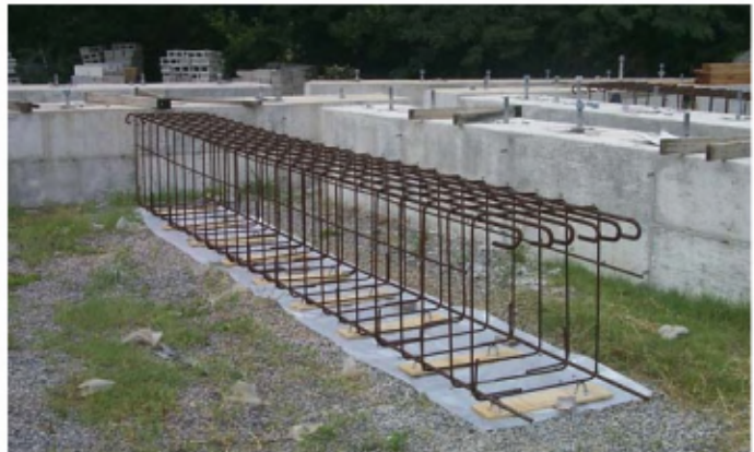
FIGURE 1 Reinforcing cage
